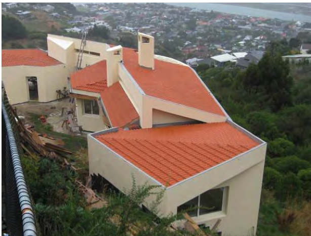
Plan irregularity increases the risk of damage.
