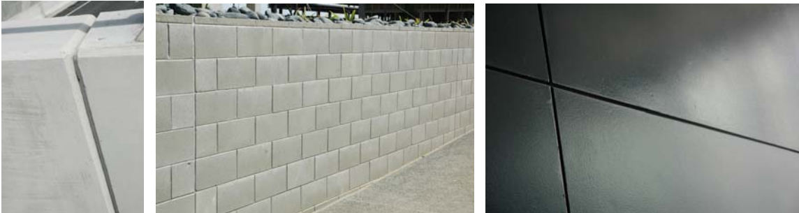
Perimeter relief using GIB® Goldline™ Tape-On Trims
