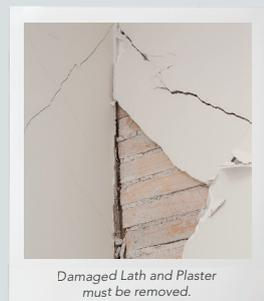
Damaged Lath and Plaster must be removed.
