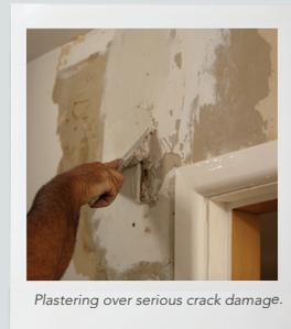
Plastering over serious crack damage.
