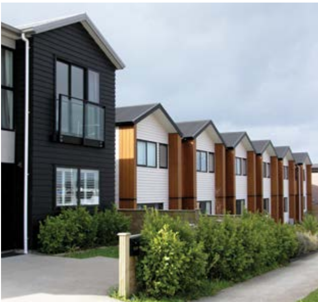
FIGURE 4: IT Barrier Systems are ideal for Terrace Homes. The central barrier remains attached to the non-fire side. Loadbearing members of the fire-affected unit can fail.
