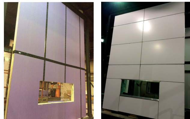
ABOVE: Preparation for the fire test with GIB Weatherline® lining (left) and with cladding (right).
