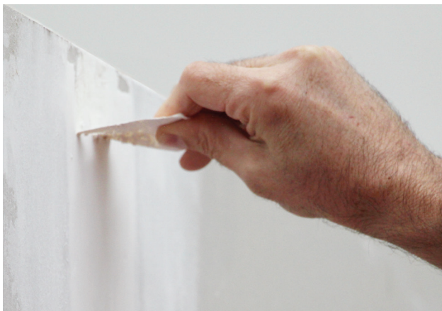
ABOVE: Paper tape pulled out of joint to check adhesion.
