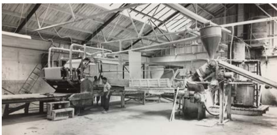
TOP LEFT: 1930 th – There are big improvements – the wallboard is now cut at its required length before going to the drier. The edges are already sealed so that no further trimming is needed. BELOW: Early wallboard production process.
