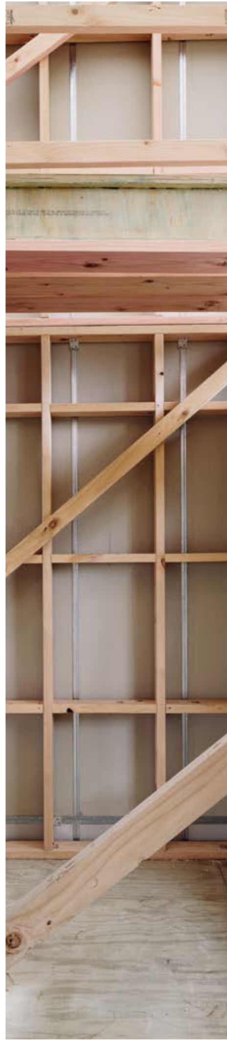
ABOVE: Example of a wall with a two way Fire Resistance Rating (FRR) – double timber frame with GIB Barrierline® central barrier. RIGHT: GIB Barrierline® installed as part of the GIB® Intertency Barrier system.
