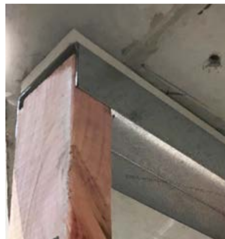
FAR LEFT: Figure 1 - Test specimens under construction at the UoC. LEFT TOP AND BOTTOM: Figure 3 - Partition framing using timber studs in metal tracks.
