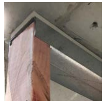
LEFT: Figure 1 - Test specimens under construction at the UoC. RIGHT TOP AND BOTTOM: Figure 3 - Partition framing using timber studs in metal tracks.
