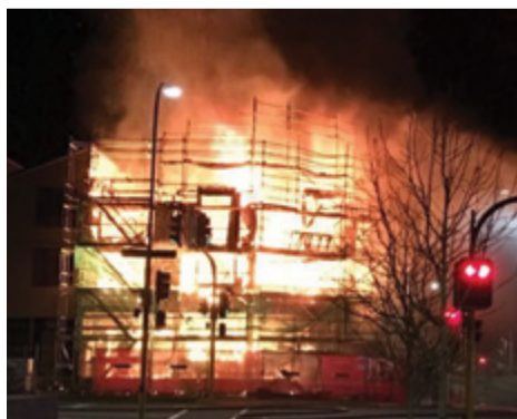
ABOVE: Figure 1, Hobsonville Point Fire, September 2017
