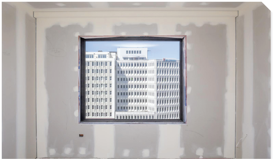
End wall of bedroom showing control/relief joints around perimeter
