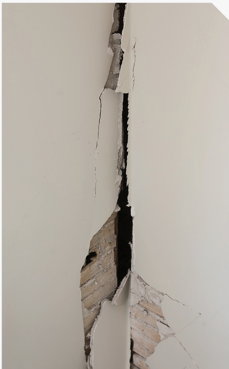
Repeat damage to cosmetic overlay
