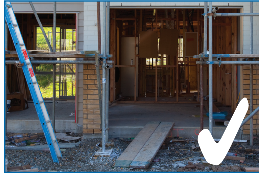
No obstructions to the site
