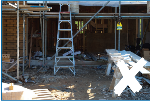
Scaffolding obstructing the building access
