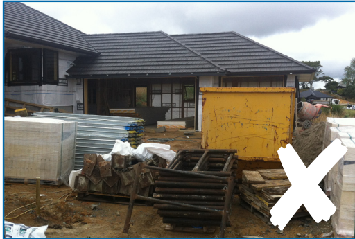
No clear access to site
