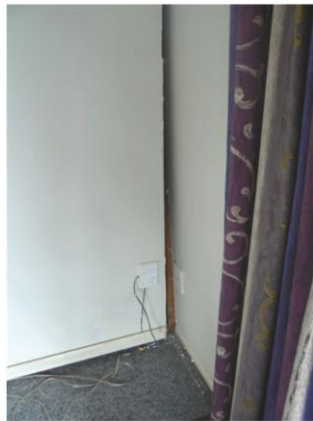
Lining detached from the framing requiring replacement of the bracing element.
