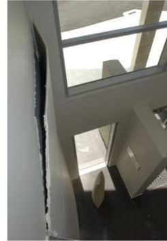
Significant sheet fracture
