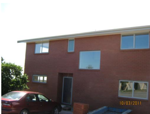
Building inspector's Mt Pleasant home under construction lost some of its brick veneer, but performed well supported by gypsum plasterboard bracing systems.
