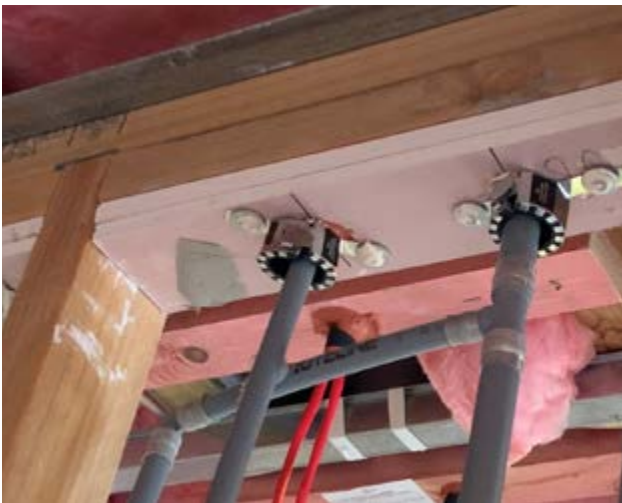
FIGURE 12: Proprietary Penetration Seals where Services pass through the Top Plate Examples of services fire-stopped using tested systems installed below the double top plate
