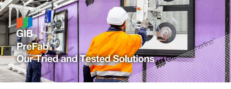
Panellised construction, an element of prefabrication, has become a method by which we can deliver more buildings in New Zealand while not being affected by weather, adverse conditions or the lack of daylight hours. Building in a controlled environment such as a factory enables faster delivery of a semi-finished product to site come rain, hail or shine – enabling quicker installation and faster overall project completion.
