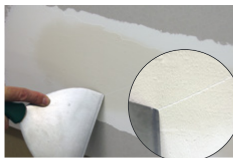
FIGURE 3: A scratch in a properly set basecoat is only super-visual and indicates it is hard.
