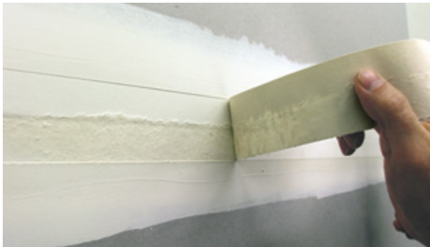
FIGURE 5: Inadequate compound under the tape and the tape can be removed relatively clean and easily.
