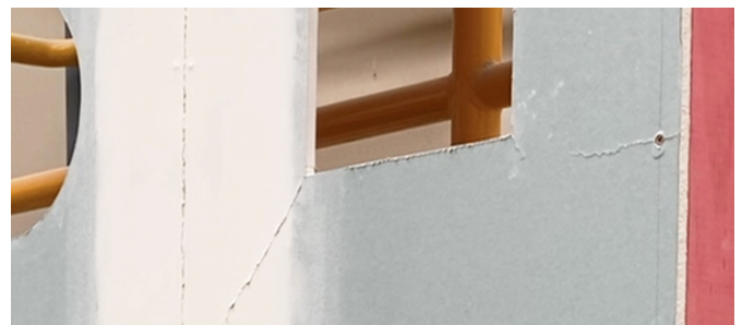
Figure 3: A close up of cracks after racking.
