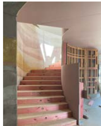
Curved GIB® plasterboard walls, (images by Avail Pacific Ltd)
